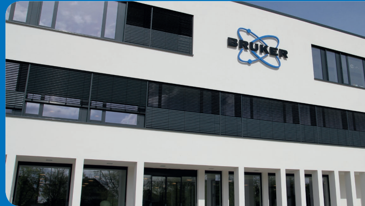
Bruker facility in Karlsruhe
